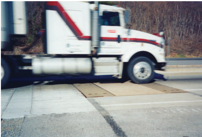
Field testing of the Strongwell deck in a truck weigh station near Troutville, Virginia, showed no signs of deterioration after 1,200,000 trucks. The second FRP deck at the Troutville test bed was subjected to 5,000,000 trucks before its removal in December 2002. Each truck represents three loading cycles.
